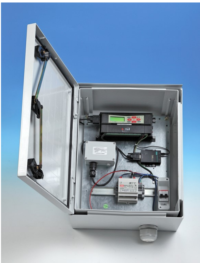
IP66 enclosure for fix monitoring applications
